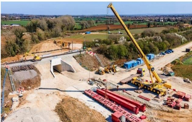
During a 100-hour railway closure between 2 and 5 April, the railway embankment was removed and two prefabricated structures - a steel underbridge and a concrete underpass with a combined weight of 2,200 tonnes - were inserted using remote-controlled transport.
